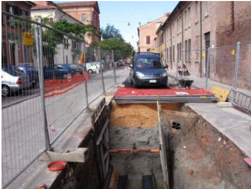
La trincea in via Scandiana
